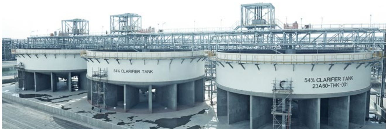
Phosphoric acid clarifiers, 30 m in diameter
