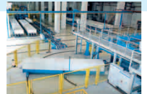
Two automated baling lines are installed at the mill, representing the newest generation of ANDRITZ bale finishing equipment in the world. Each line is designed for a capacity of 300 bales per hour. ▶
