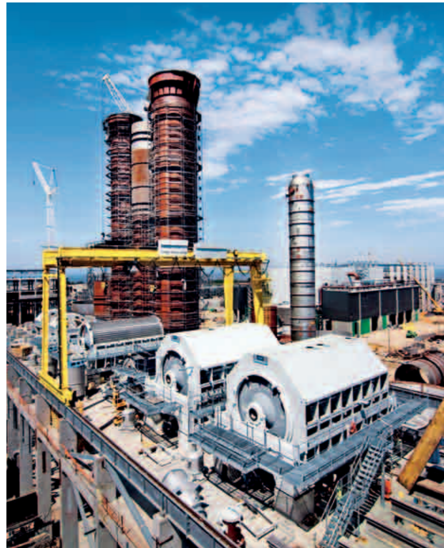
◀ DD washers on the fiberline are being set in place. The bleaching towers are in the background.
