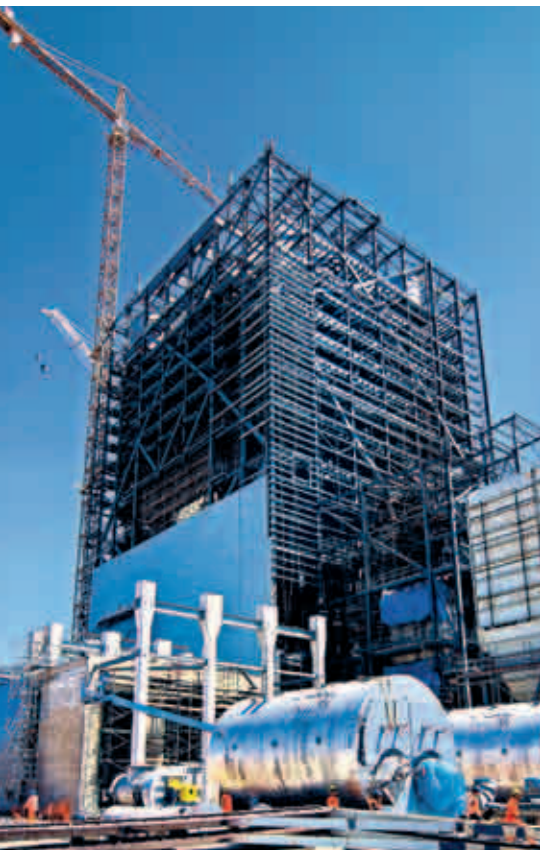
▲ Work proceeds on the recovery boiler (main structure) and power boiler (lower left).
