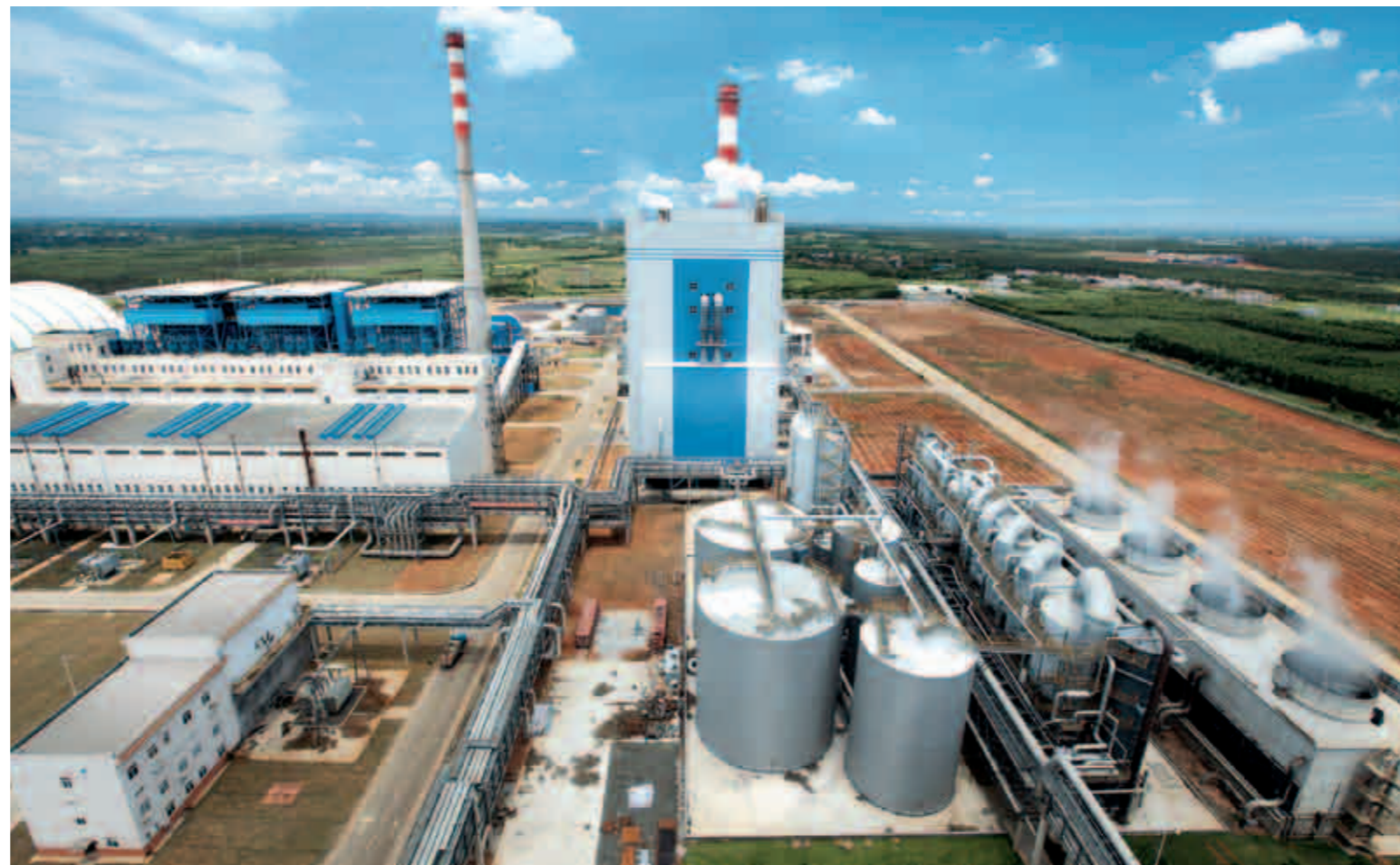
◀ View of the evaporation plant (foreground) and recovery boiler. Black liquor is concentrated to 80% dry solids before being fired in the 4,450 tds/d recovery boiler.
