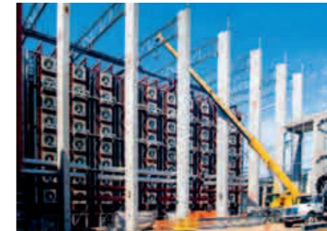
▲ A construction crane lifts sections of the airborne pulp dryer into place.
